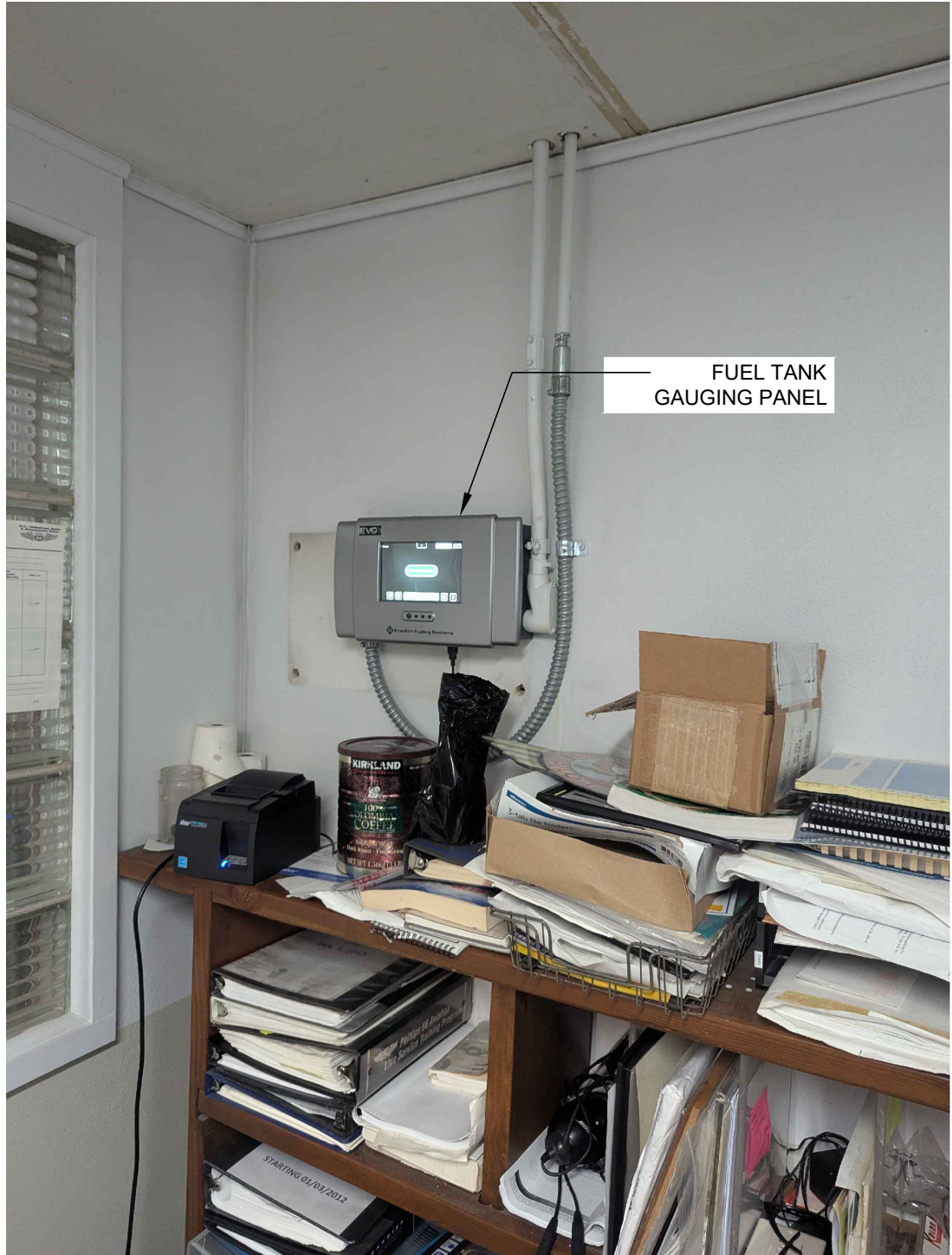
3 FUEL TANK GAUGING PANEL e1.04 NO SCALE
