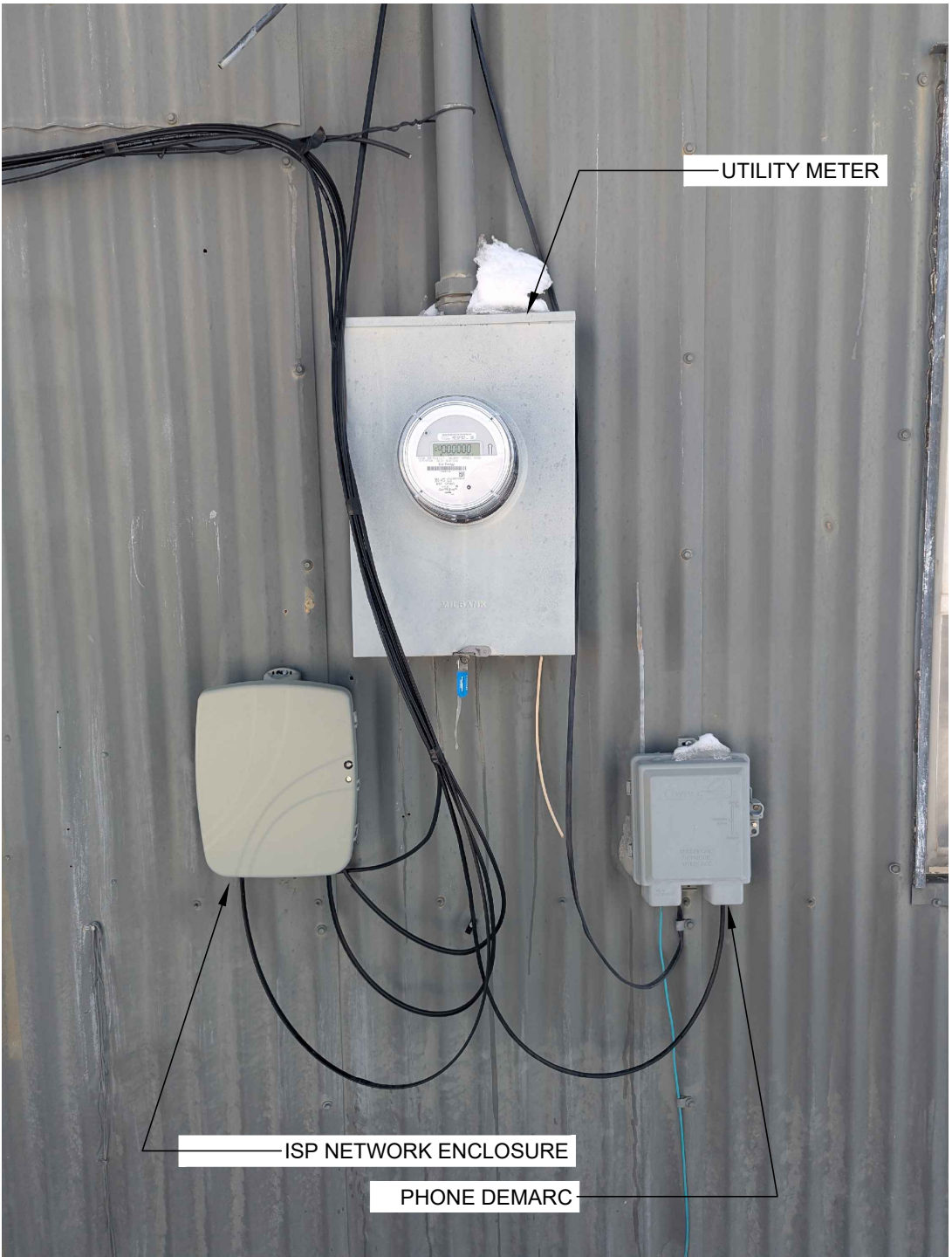
4 ISP NETWORK ENCLOSURE e1.04 NO SCALE
