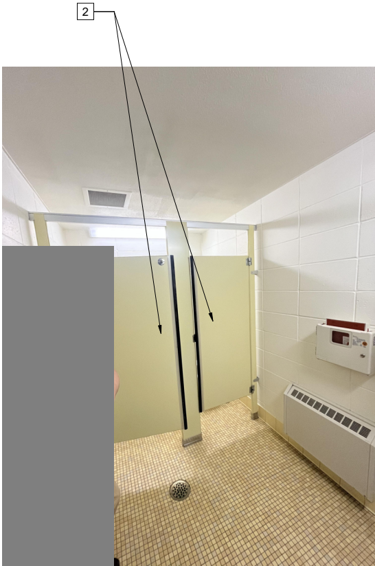
2 WOMEN'S BATHROOM LOOKING EAST A0D105
