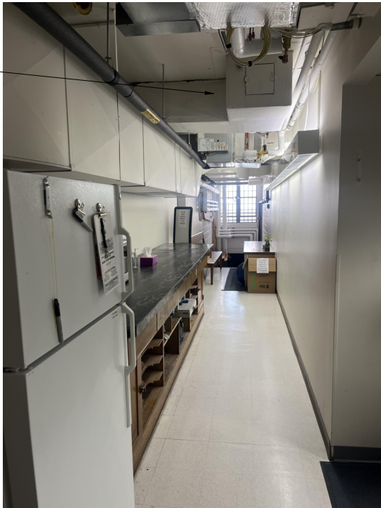
6 IT CORRIDOR LOOKING NORTH A0D103
