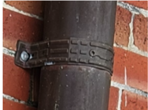
Figure 1 - Richland Center Existing Downspout Strap (Universal Conductor Band)
